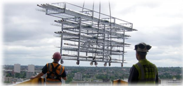
Figure 5 Prefabricated conduit system being lifted into a building
