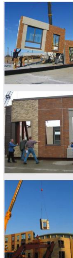
Figure 4 Construction of prefabricated, load-bearing wall sections
